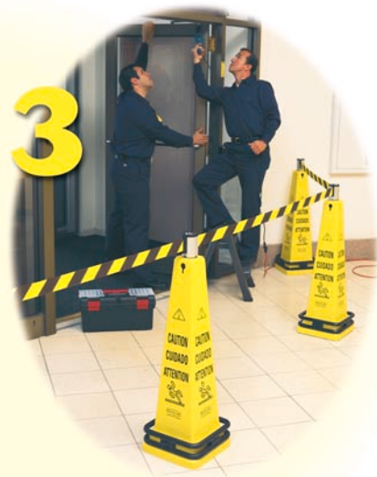
Barricade System safely redirects patrons around work areas and ensures worker productivity.
